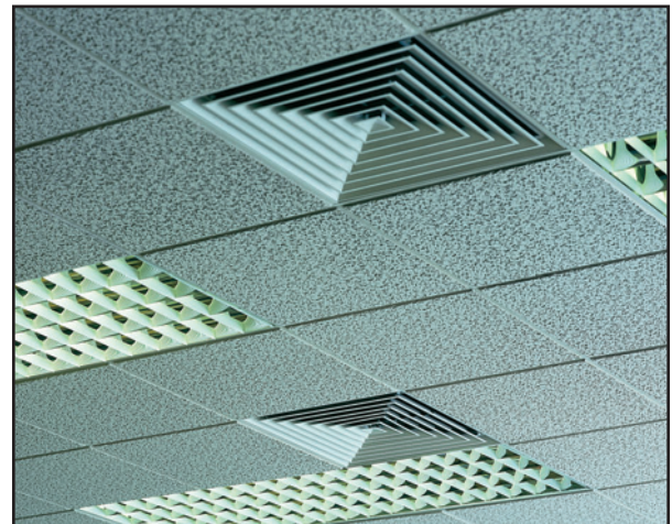
Louvre face diffusers in a typical installation
