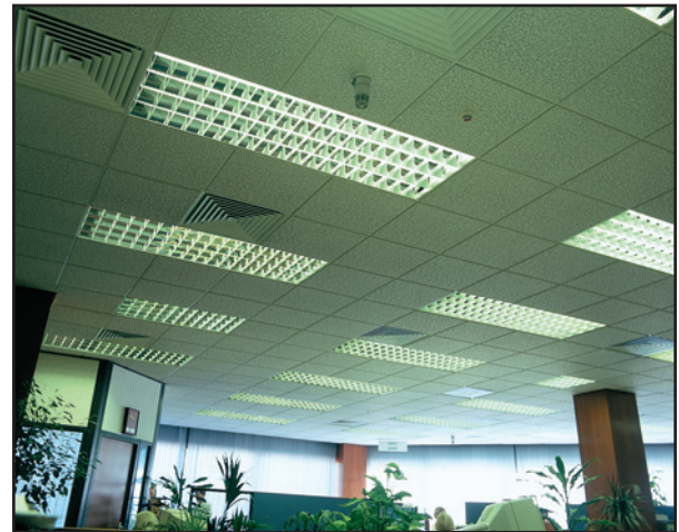
Louvre face diffusers in a typical installation
